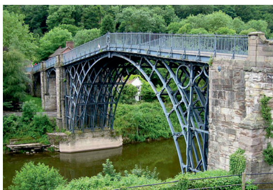
Fig. 2. The first cast iron bridge built in 1779 in England across Severn river
